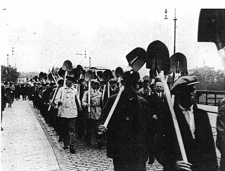
9.26 Army of unemployed as construction workers for the Frankfurt Autobahn.
