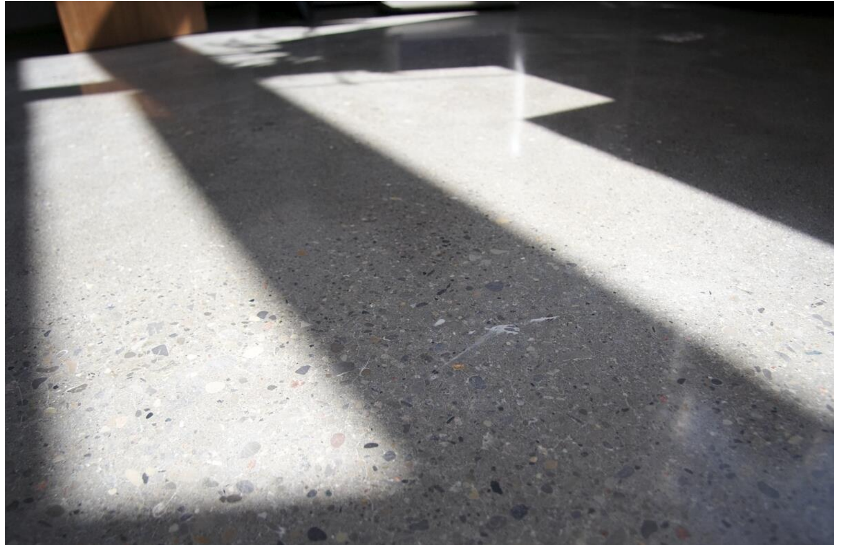
Moving in-002744; Polished concrete floors. Photo: Evan Borgstrom @ Flickr
