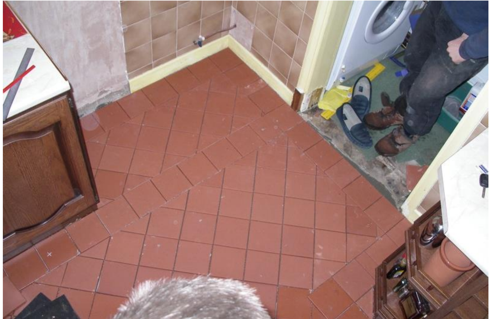
The kitchen tiling is done! – photo by Jonathan @ Flickr
