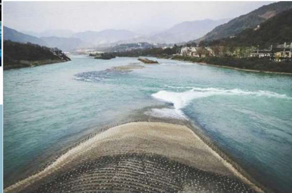
The 'Fish Mouth' levee. Part of the Dujiangyan irrigation system. (CC0)
