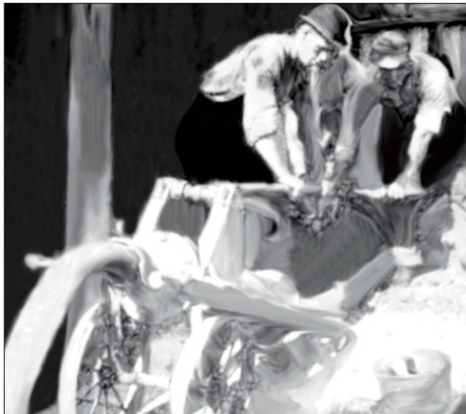
Photo II.6. "Made in Baltimore." An odorless excavator, used in cities to pump out vaults and cesspools. The odorless excavator was actually a Paris innovation. Source: Survey , 1911.
