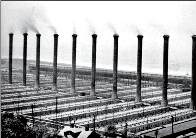
Photo v.3. World's largest concentration of beehive ovens—Jones & Laughlin Iron & Steel Company, located in “Hazelwood,” Pittsburgh. Source: Guy C. Whidden and Wilfred H. Schoff, Pennsylvania and Its Manifold Activities (Philadelphia, 1912).
