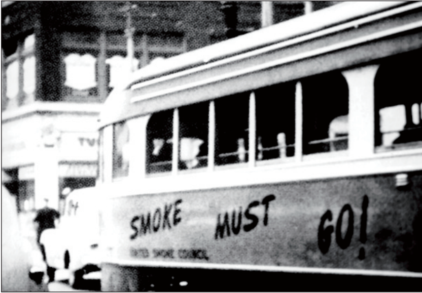
Photo III.5. Pittsburgh Smoke Control Campaign, 1941. Source: Allegheny Conference on Community Development.
