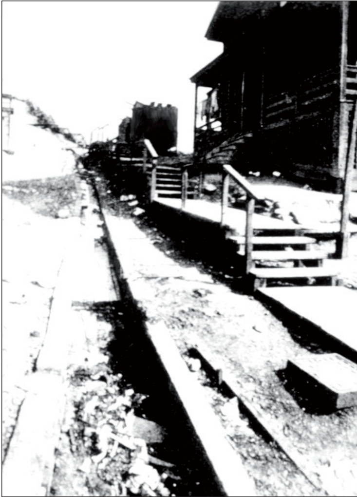
Photo II.7. An open sewer in Pittsburgh. Source: Paul Underwood Kellogg (ed.), The Pittsburgh District: Civic Frontage, The Pittsburgh Survey (New York: Survey Associates, 1914).
