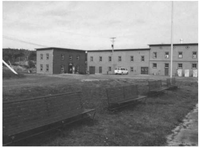
Figure 1.6. A view toward the east, showing the Disinfection Building and the Carpentry and Plumbing Building (now the Visitor Center and gift shop) at the left. Built in 1892 on the north end of the western wharf, the Disinfection Building housed three disinfection chambers and, eventually, showers. The south wing was erected in 1915; the north, in 1927. The Disinfection Building has been restored to its 1927 appearance; it is the first place modern visitors enter.
