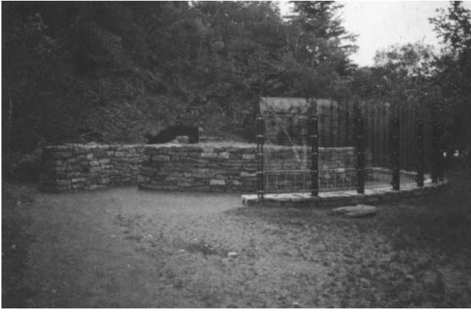
Figure 1.18. The new Irish Memorial is tucked against the hillside, just southwest of the Doctors' Memorial and above the Irish Cemetery. The stone structure in the center is framed by glass panels etched with the names of the dead from the epidemic years.
