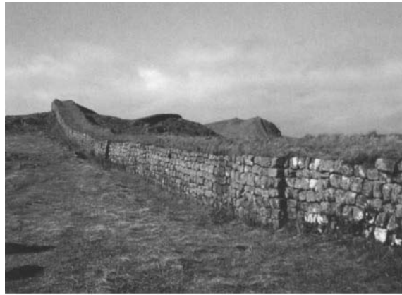
Clayton's Wall, near Steel Rigg. Many segments of Hadrian's Wall could be considered reconstructions. For example, in some places much of the wall was mined for building stone in the post-Roman era. The extensive sections of Clayton's Wall reconstructed in the nineteenth century (followed by similar conservation in the twentieth century) consist of a core of excavated and reassembled Roman-era dry-laid wall with nineteenth-century course layered on the top. Few, if any, truly authentic segments of exposed wall survive. Photo: Marta de la Torre
