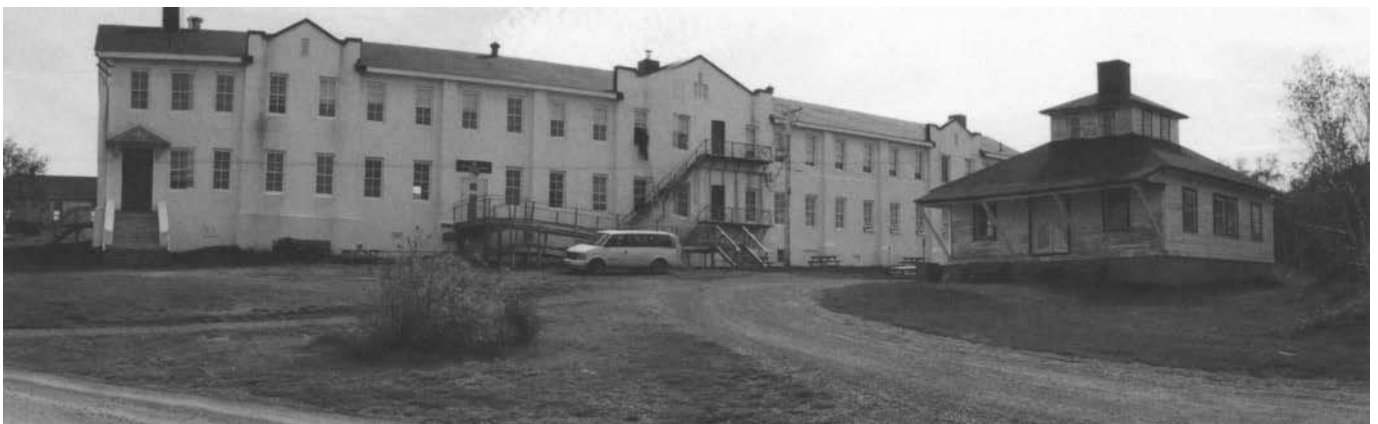
Figure 1.14. The Third Class Hotel, built in 1914, is the largest of the three hotels, designed to hold 140 beds in its fifty-two rooms. Built of concrete, it included kitchens and dining areas at either end of each floor of the building, with living quarters in the center. While it offered close quarters and little privacy, it was fitted with electricity and central
