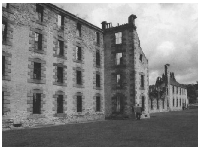
Figure 3.6. The penitentiary building, the largest and most prominent structure from the convict period. Photo: Marta de la Torre
