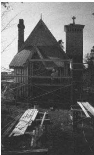
Figure 1.10. The Anglican Chapel (location 11, fig. 1.3). Built in 1877–78, the Anglican Chapel was made of wood and set on masonry pillars. It was intended for the use of the staff and residents of the island, not for the immigrants. In order to preserve the structure's largely original appearance and to stop leaks, the pillars are being reinforced; a moisture barrier is being placed between the interior walls and the board-and-batten exterior skin; and the tin roof is being repaired.
