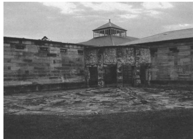
Figure 3.11. The exercise yards of the Separate Prison. The exercise yards lie in ruin today. Conservation and interpretation plans call for partial reconstruction of these yards. Photo: Marta de la Torre
