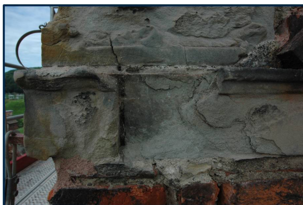
Fig. 2 Gdańsk, sandstone Gotland, architectonic detail - black crusts formed on the stone surface, cracking, peeling off, detached fragments, granular disintegration (J. W. Łukaszewicz)
