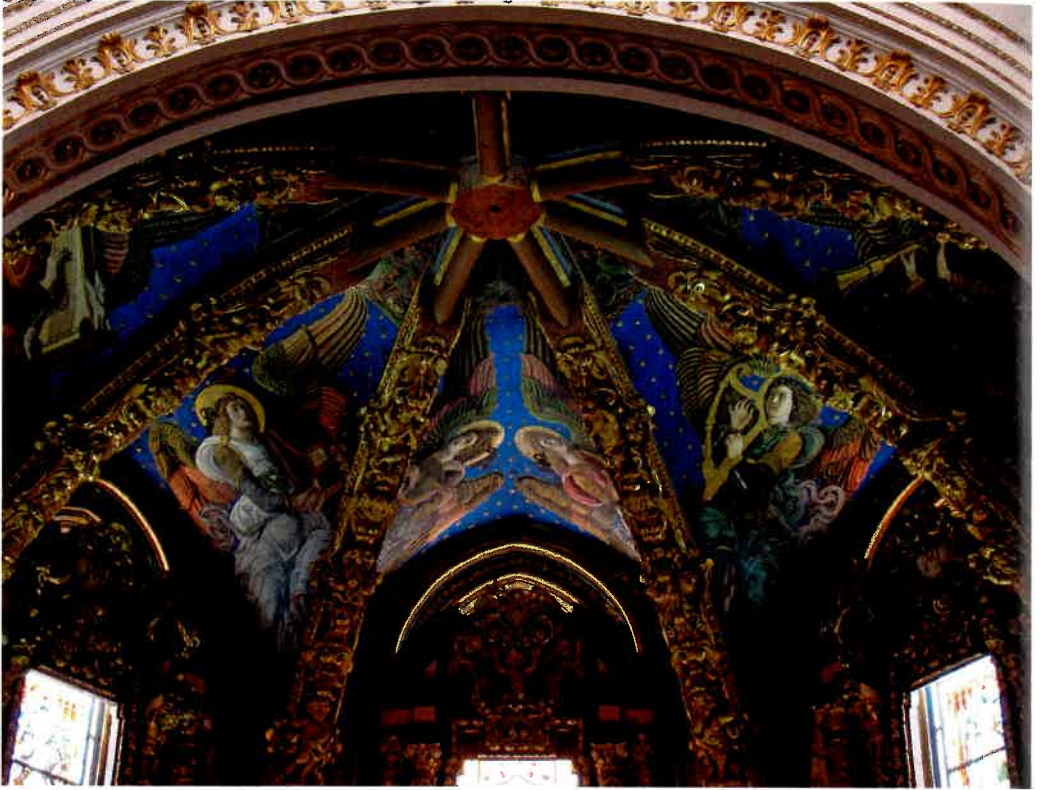
Figure 7.2 Detail of the half-dome of the chancel of the cathedral of Valencia. The photo shows the Gothic ceiling with the Renaissance paintings, the central ends of the Gothic ribs, the Baroque ornaments in the outer ends of the ribs and the modern, minimalist cornerstone: a creative, truly innovative blend of elements from different times and styles. (Photo © Salvador Muñoz Viñas.)
