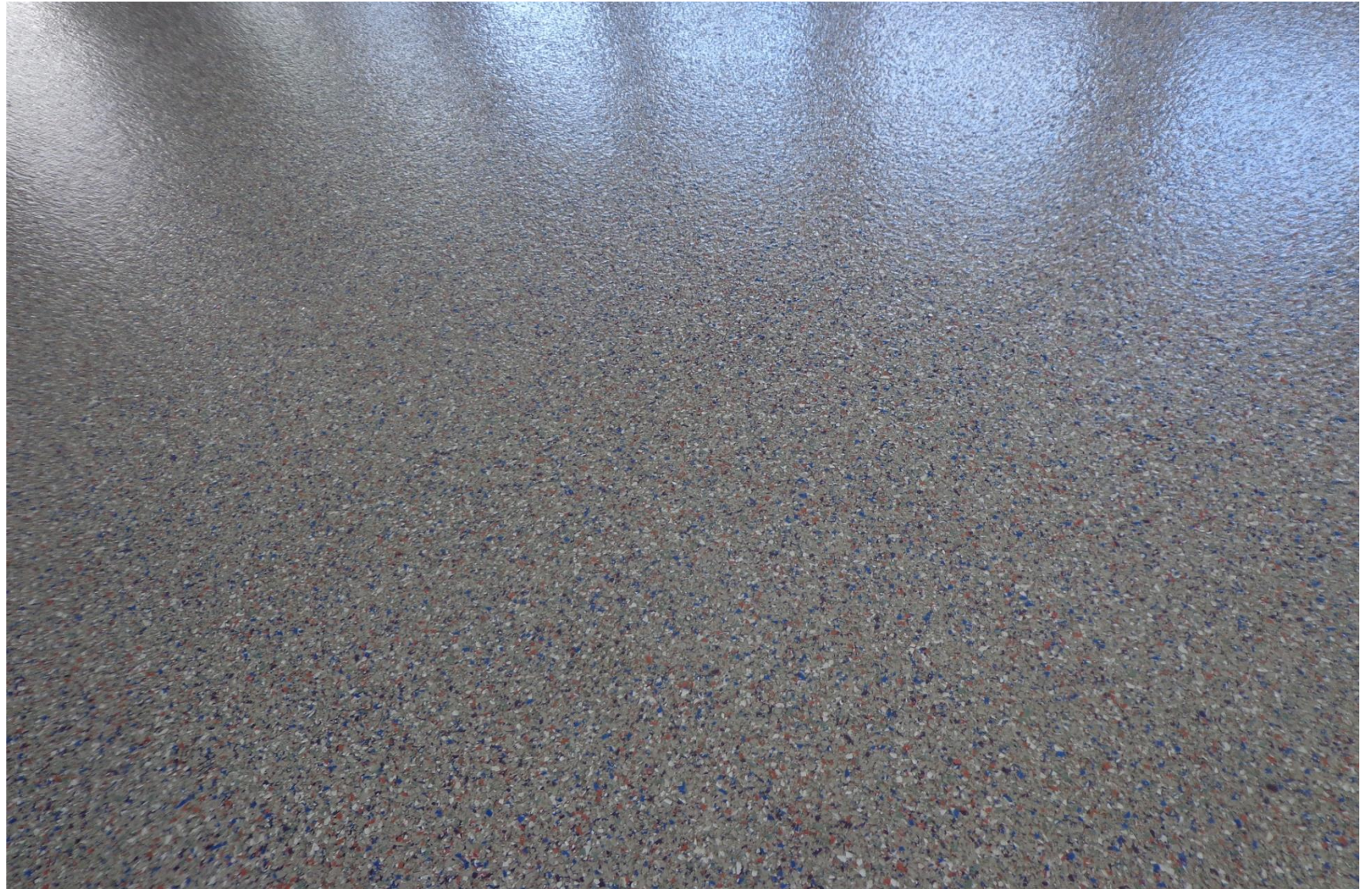
"Muliti Chip Custom Blended Epoxy Coating" by Decorative Concrete King @ Flickr
