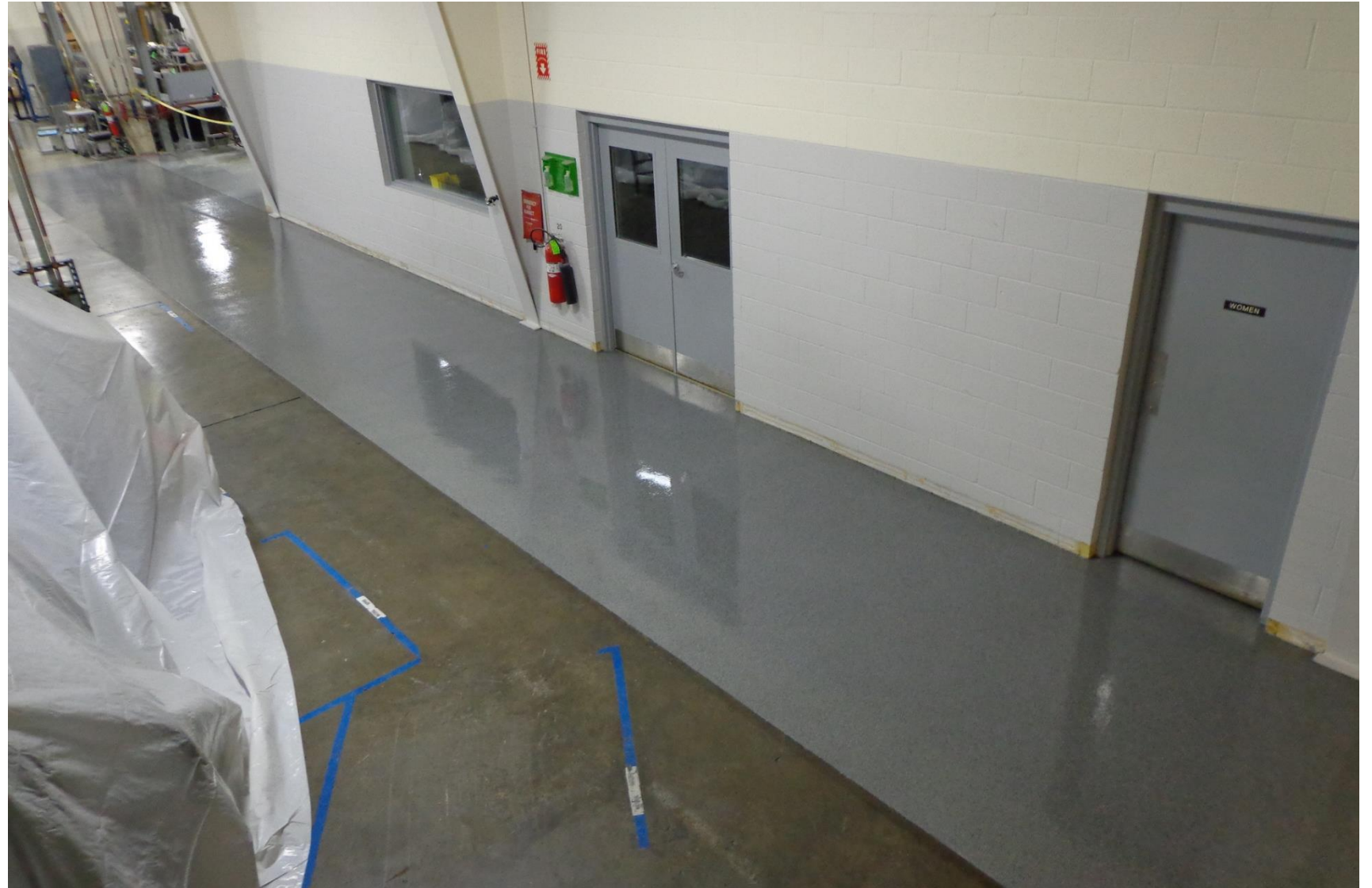
"After Pic Of Epoxy Flooring Taken From Stairs" by Decorative Concrete King @ Flickr
