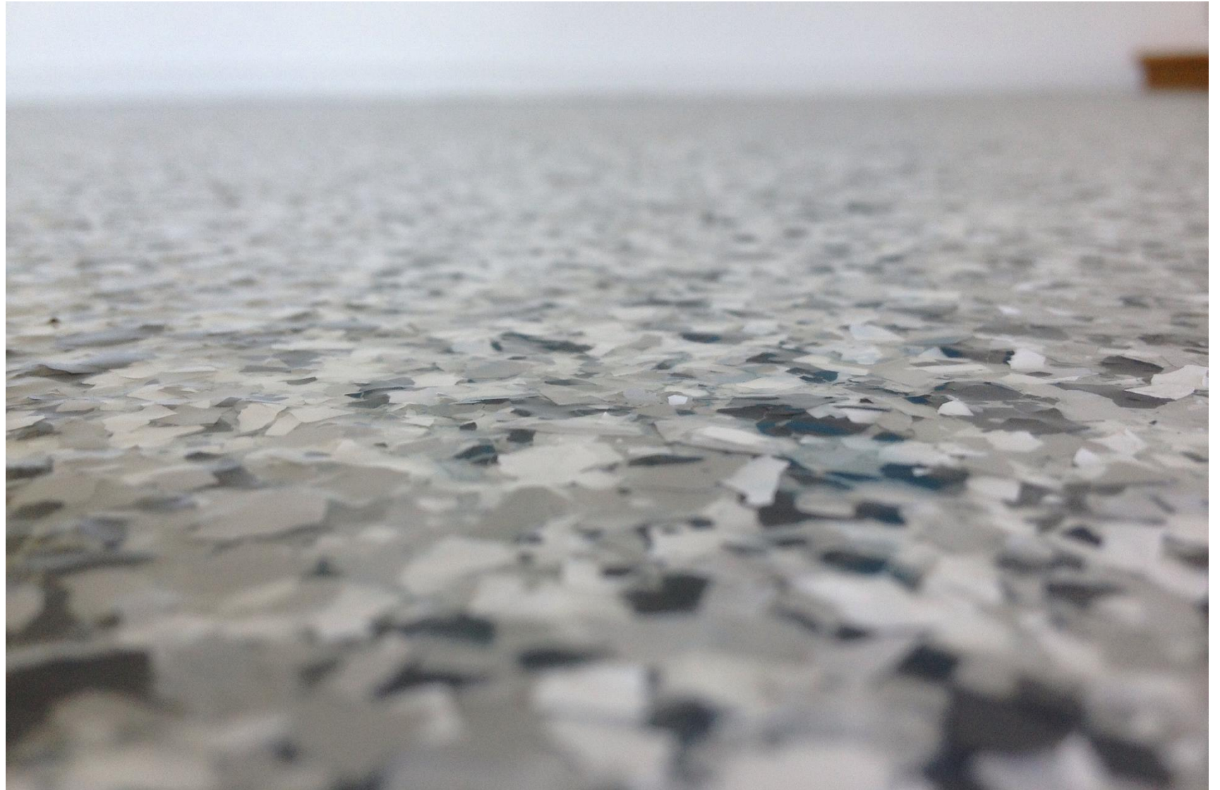
"Vinyl chip epoxy garage floor in Charlottesville, VA" by Tim Seay @ Flickr
