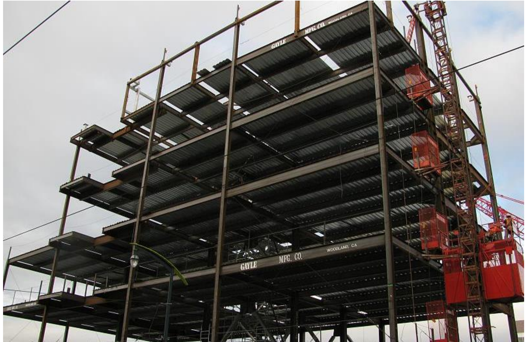
steel frame of building 1. Photo: Steven Damron @ Flickr
