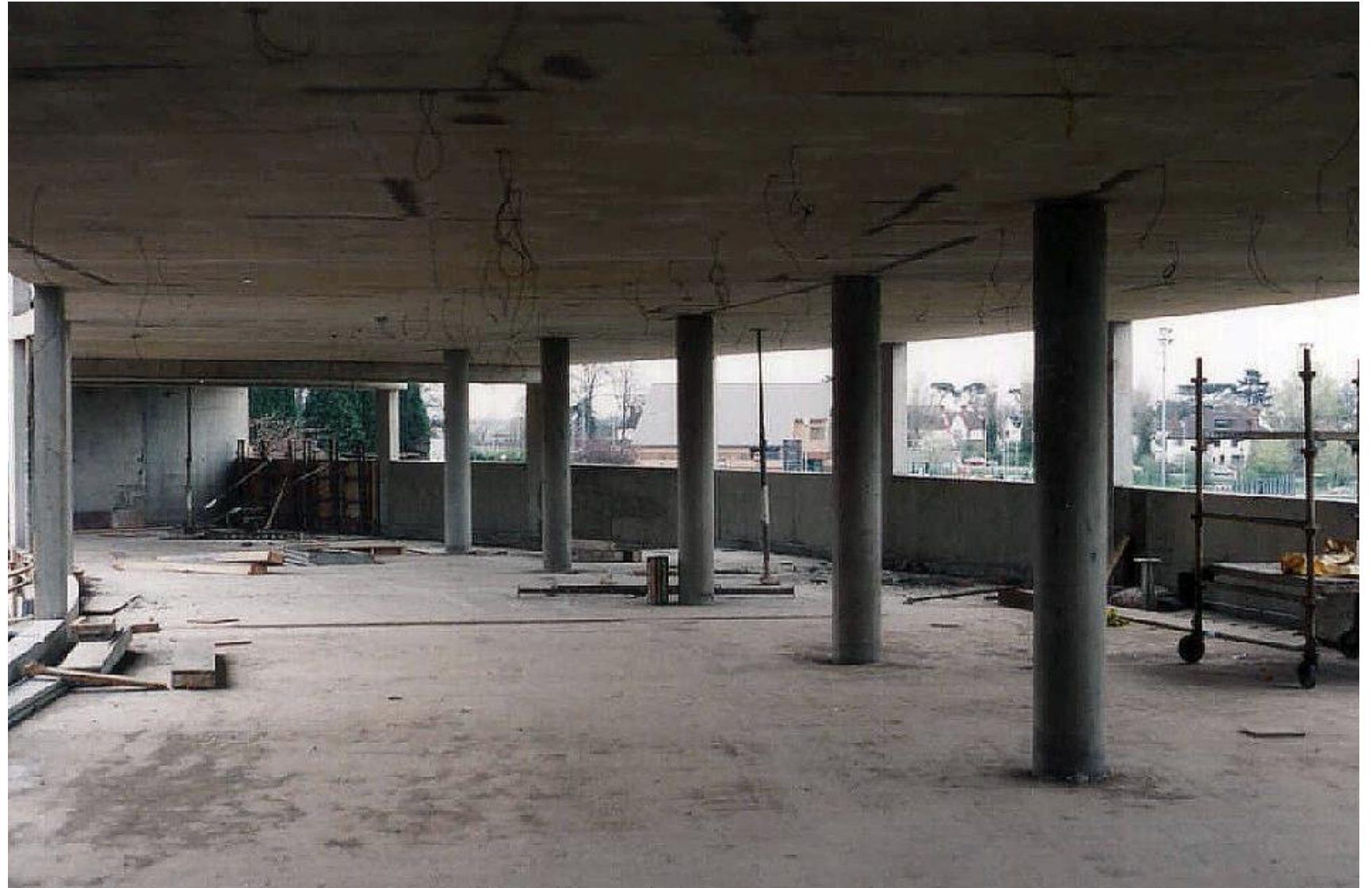
Insitu concrete suspended slab. Photo: Loughborough University @ Flickr: © luf:240200:l0004
