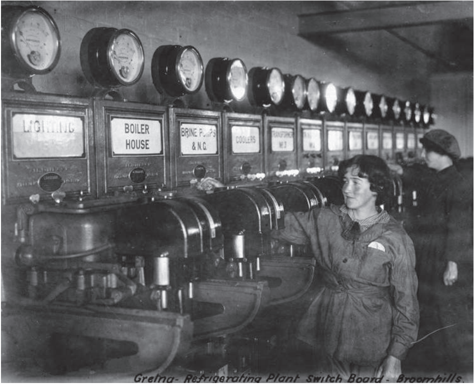
Gretna - Refrigerating Plant Switch Board - Broomhills.
