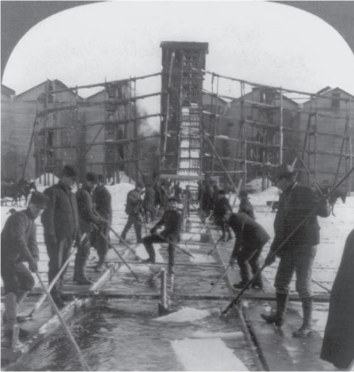
Blocks of ice being guided to the icehouse elevator, Keystone View Company, Conneaut Lake, Pennsylvania, 1907.
