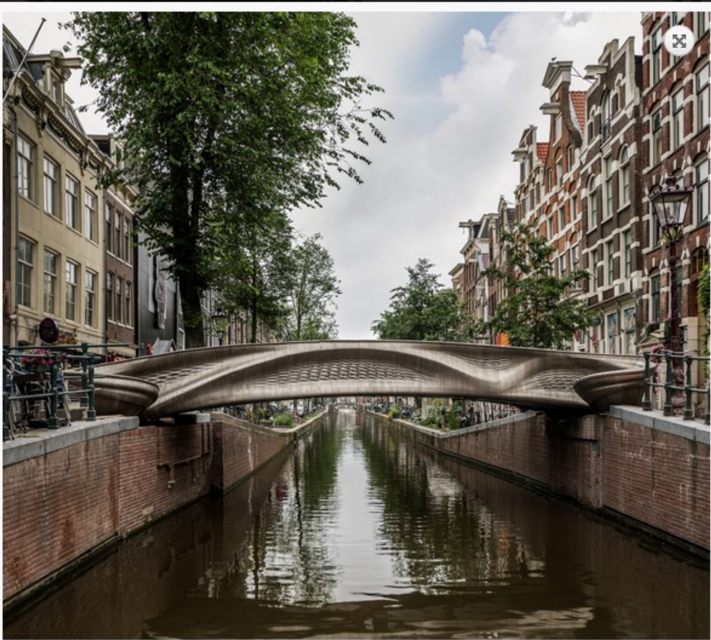
MX3D's 3D-printed pedestrian bridge
