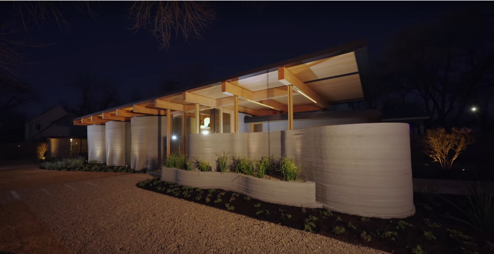
ICON's House Zero - 3D-printed Home Pushing Boundaries of Sustainable Architecture & Design
